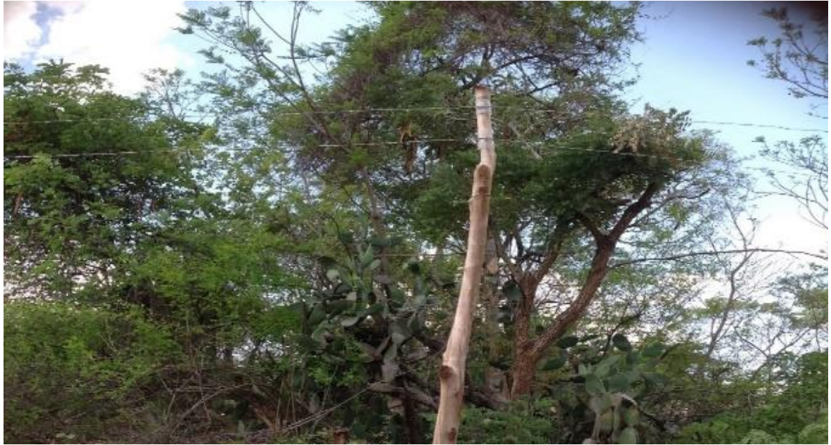
Illegal electricity connection: Auditor – December 03, 2021
